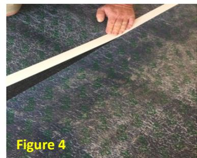
2. Cover the entire floor area to be fitted with Ustik® underlay, leaving an expansion gap between the Ustik underlay and the perimeter wall of approximately 3mm, as this will allow for expansion and contractions of this floating floor system.
