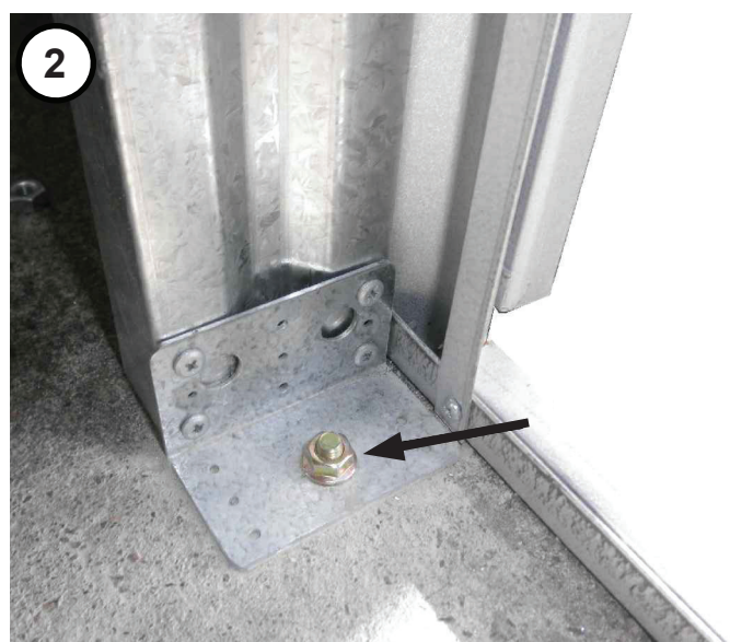
Door stud have a single anchor through a BKT17. Fixed by four tek screws.
