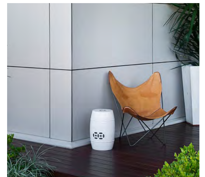
Matrix™ Cladding Horizontal layout with joints painted black.
