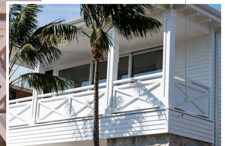
Diagonal pattern in balustrade
