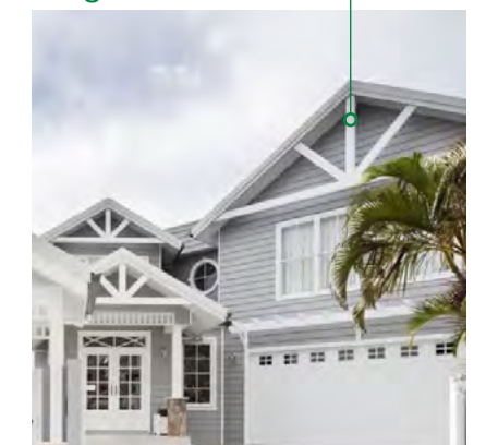
Open gable with King Post trusses
